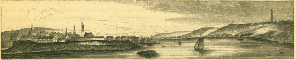
NEW LONDON HARBOR, LOOKING NORTH. 2
