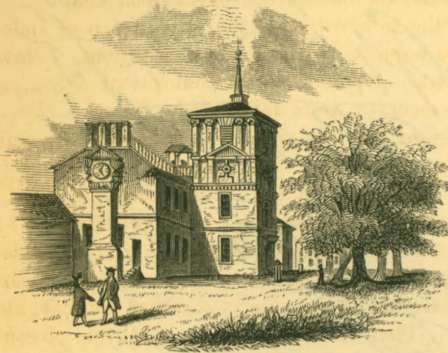
WALNUT STREET FRONT OF THE STATE HOUSE IN 1776. 2
