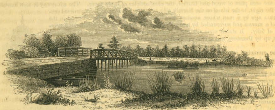
VIEW AT THE GREAT BRIDGE.
