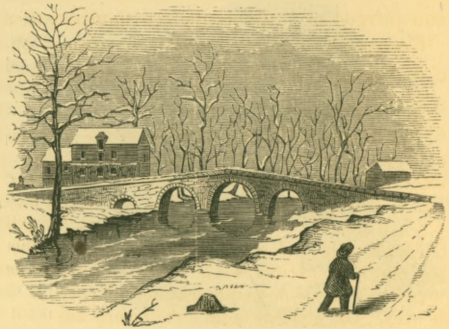
BRIDGE AT WORTH'S MILLS. 3
