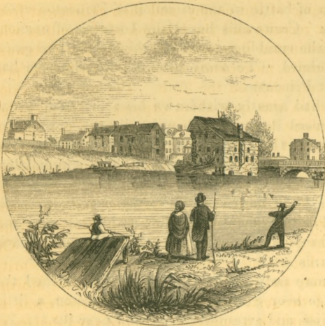
TRENTON BRIDGE AND VICINITY. 3
