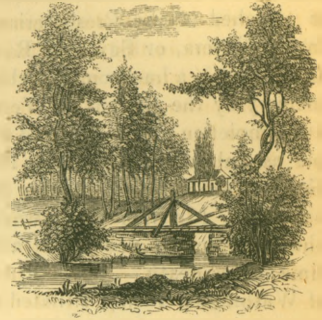
BRIDGE OVER SLEEPY HOLLOW CREEK.
