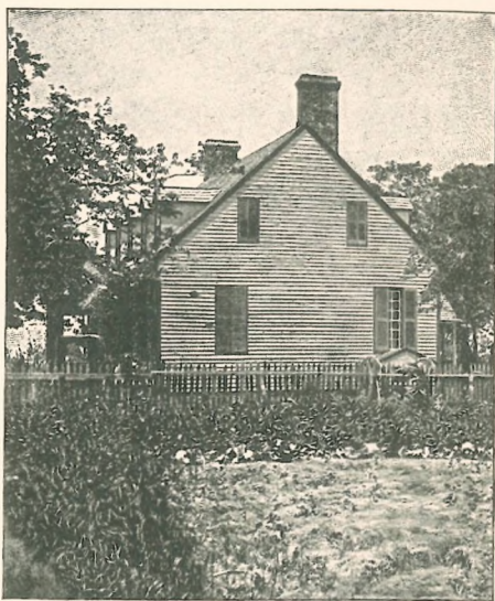
THE WEST HOUSE AT YORKTOWN (Showing the shot holes)
