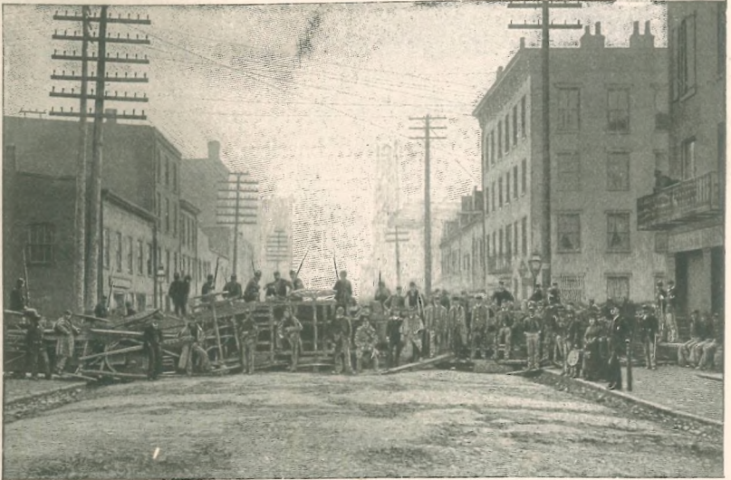
THE CINCINNATI RIOTS OF 1884 The Barricade in South Sycamore Street
