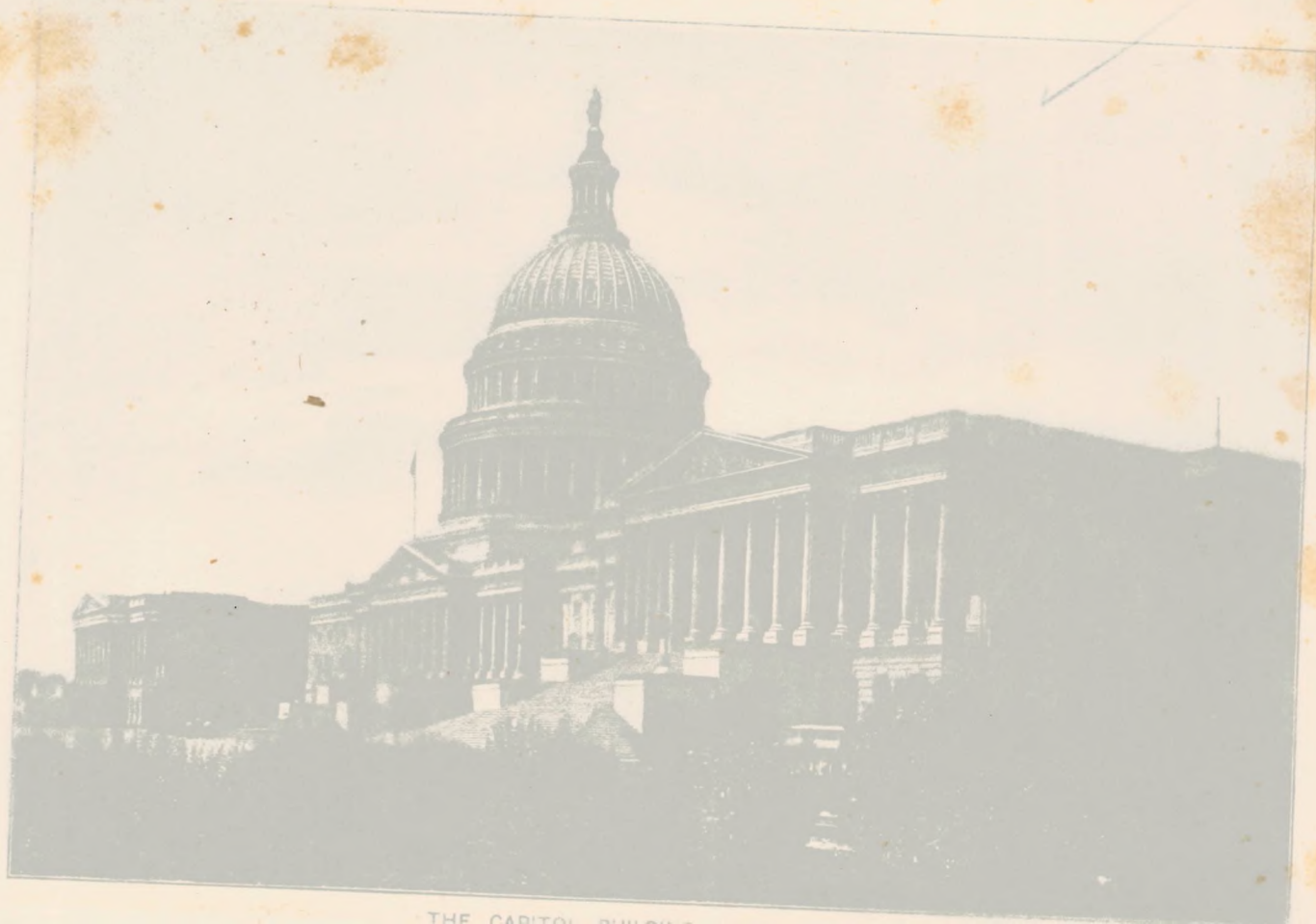
THE CAPITOL BUILDING
