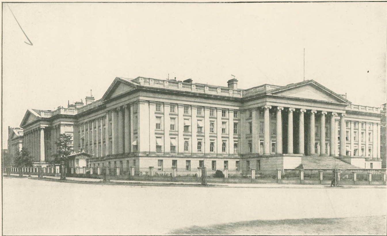
TREASURY DEPARTMENT BUILDING.
