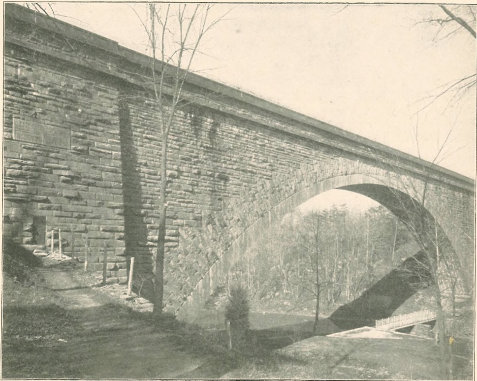
CABIN JOHN BRIDGE AND ITS FAMOUS ARCH.
