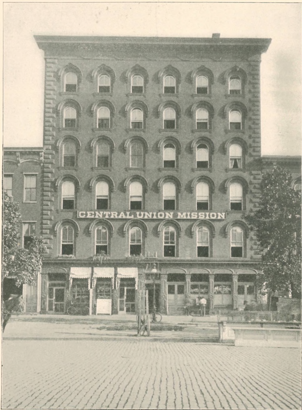
THE HOME BUILDING OF THE CENTRAL UNION MISSION.
