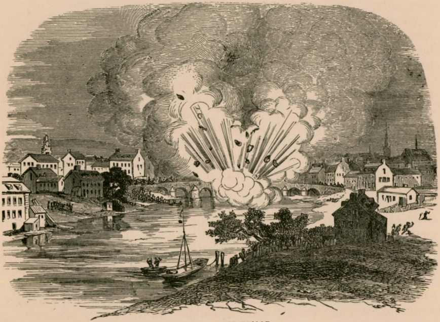
DESTRUCTION OF THE BRIDGE.
