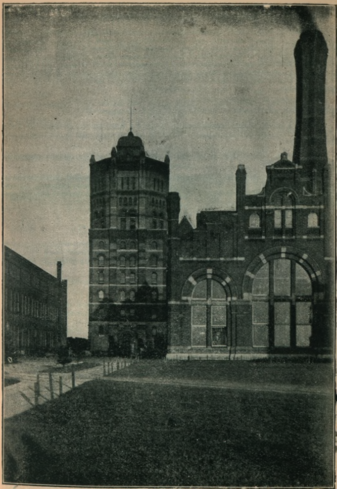
[Engraved for The Standard Guide Company.] CORLISS ENGINE HOUSE AND WATER TOWER, PULLMAN, CHICAGO. [See "Pullman,"]
