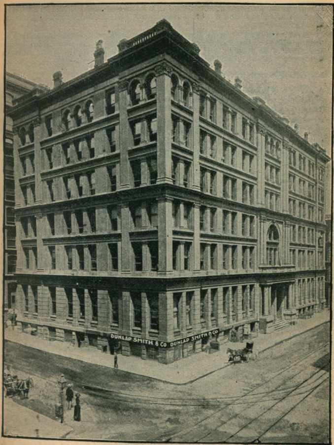
[Engraved for The Standard Guide Company.] FIRST NATIONAL BANK BUILDING. [Office of Dunlap, Smith & Co.]
