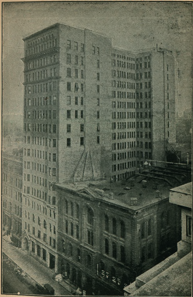
[Engraved for The Standard Guide Company.] TITLE AND TRUST BUILDING. MEAD & COE, AGTS. [See Page 196, and "Mead & Coe."]
