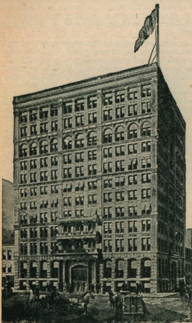
HOME INSURANCE BUILDING.—See Buildings.
